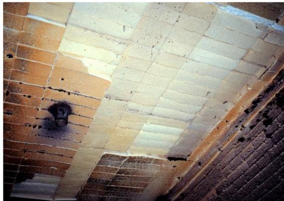
**Figure 31: Crown of Sawdust Fired Tunnel Kiln After Seven Years Showing Surface Glazing and Sheet Spalling**
