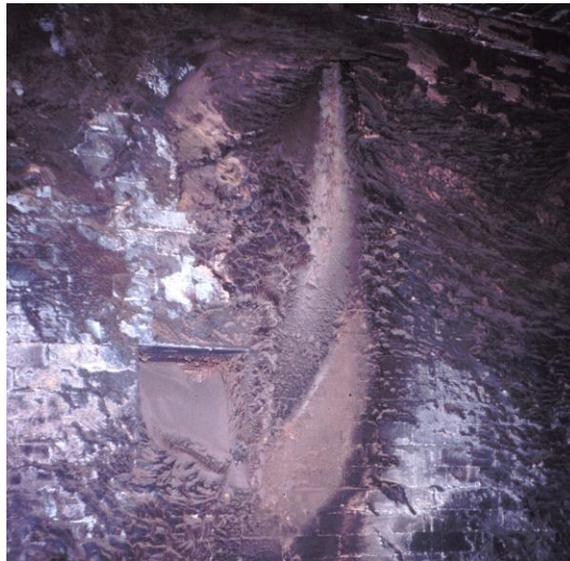
**Figure 30: Sidewall of Sawdust Fired Tunnel Kiln After Seven Years of Service**
