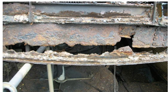
Once exposed, a floor beam may look like this.
