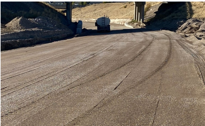
Roadway construction and site development
