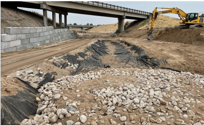
Heavy civil drainage and roadway construction
