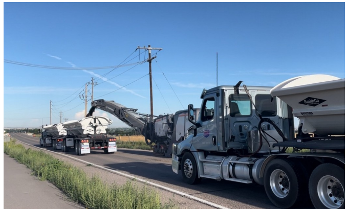
Roadway milling and paving operations
