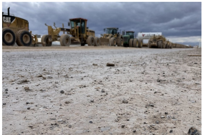
Heavy-equipment fleet support and field operations
