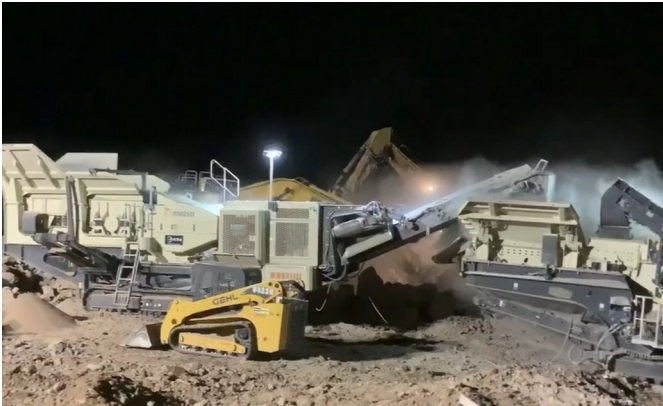
Crushing and screening operations
