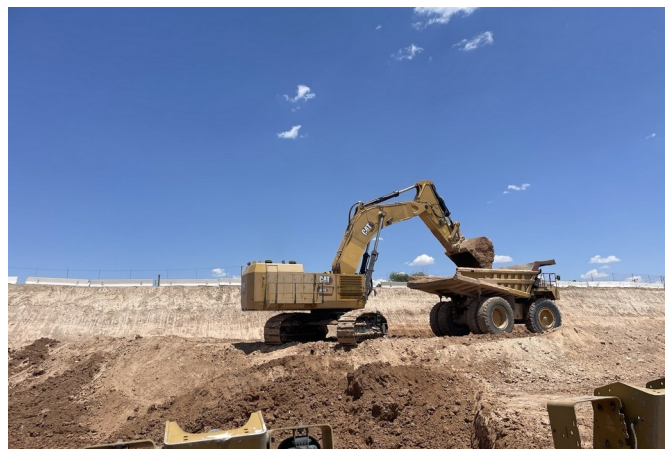
Excavator and off-road haul-truck production
