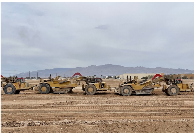
Scraper fleet operations and site development
