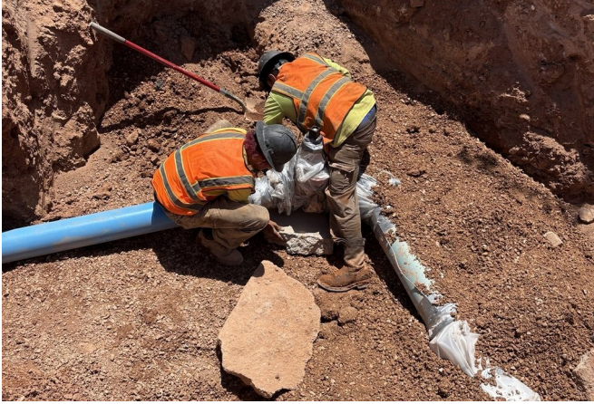
Underground utility installation and field operations
