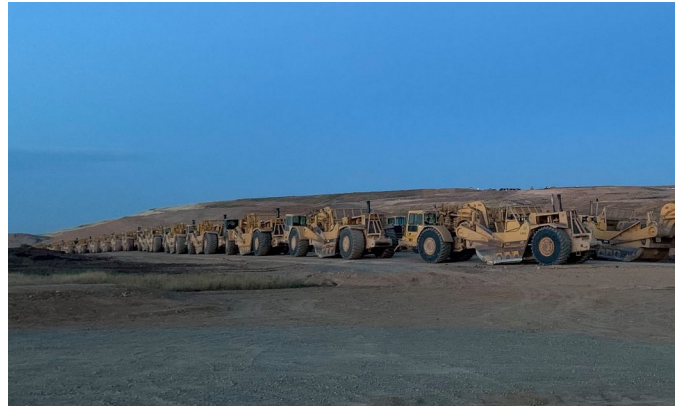
Large scraper fleet and equipment management
