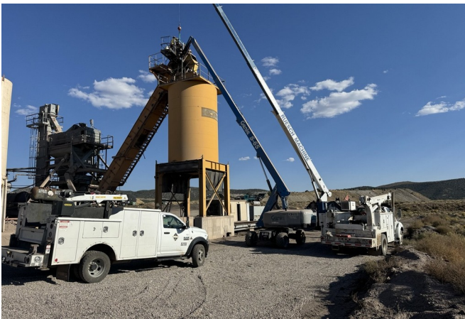
Plant maintenance, lifting, and operational support
