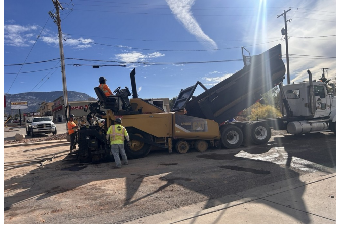
Asphalt paving operations and truck coordination
