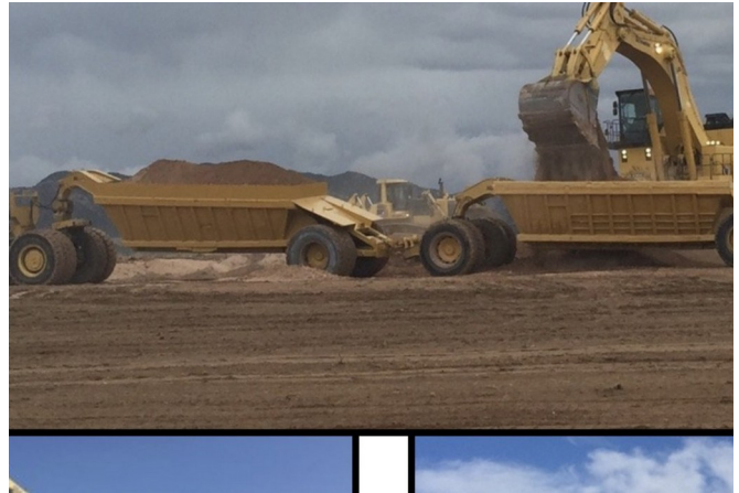
Excavator loading scraper spread - mass earthwork
