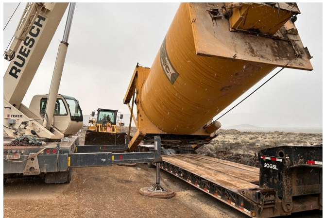
Plant equipment mobilization and heavy-lift support
