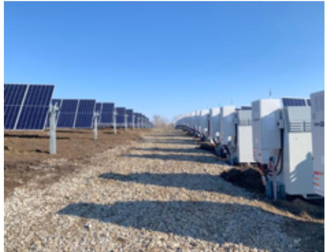
*A NEXTracker's NX Flow integrated solar-plus-storage system with DC-coupled NEM energy storage. Image: Courtesy of Ideal Energy*
