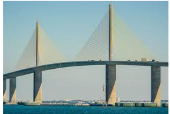
2 The Tampa Skyway Bridge
