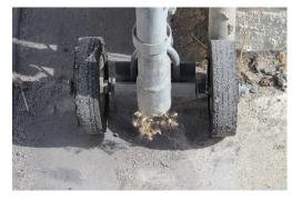
These rolling wheels take a portion of the sliding gate weight and need to be properly maintained for alignment so that the gate travels in a straight line.
