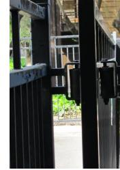
There are usually at least two components that are observed to be missing or defective regarding gate stops. One is the absence of any restricting stop component, the other are missing or broken pinch rollers that are used to guide and align the sliding gate as it opens and closes.
