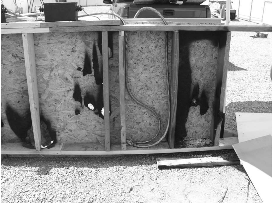
Figure 8 - Neon transformer testing burn patterns
