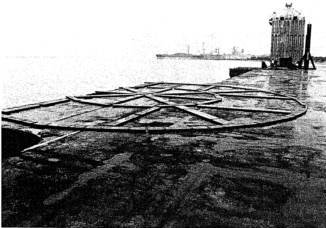
Fig. 10 - Cribbing arrangement for forward starboard column.
